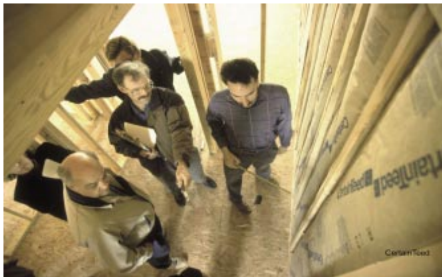
Insulation inspection - photo courtesy of Certain Teed Corporation
